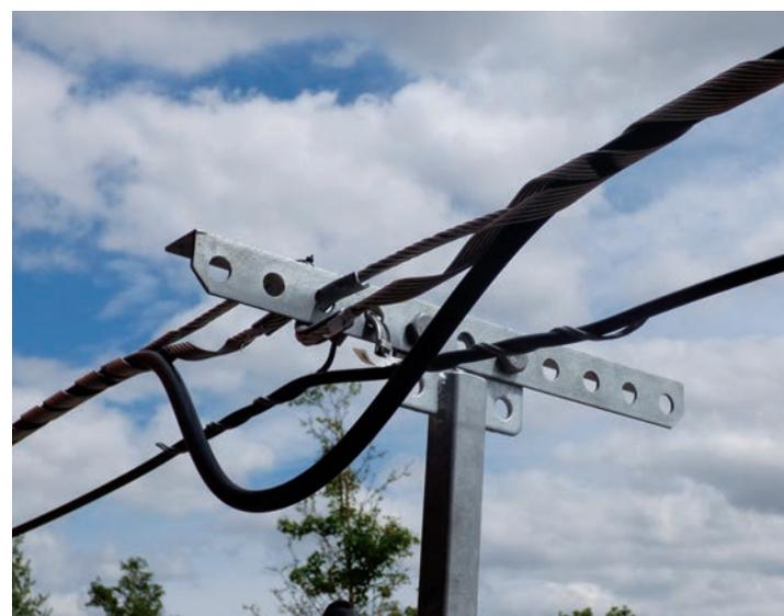
Pole extension + cross-arm with double dead-end anchoring and suspension.
