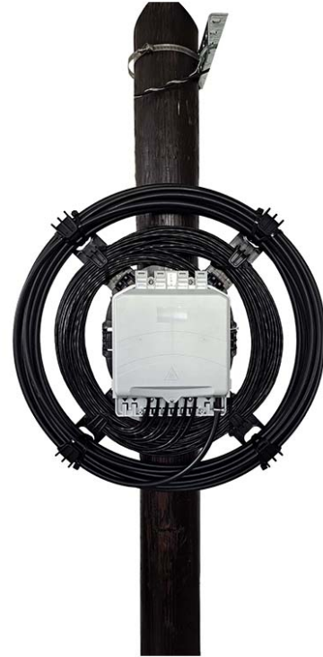
Slack Cable Storage for MAB (with an extension to 600 mm and MAB box)
